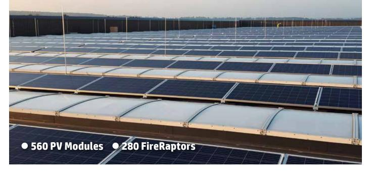
We were approached by a specialist PV installer who was seeking a solar panel rapid shutdown solution for Boeing GoldCare's 16,000sqm aviation hangar facility which housed 560 PV modules on a single-ply membrane roof at Gatwick airport in the UK.
